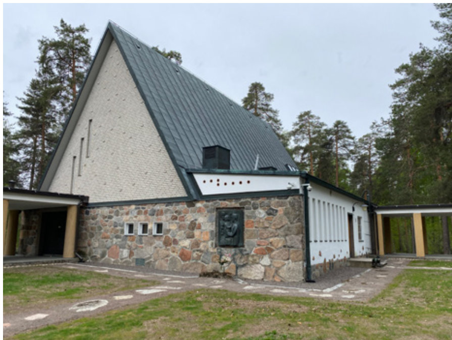
Figure 4. Boulders of local rock types has been used in the lower part of the façade of the Ristikangas Funeral Chapel. Photo: Olavi Selonen.
