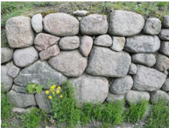
Figure 1. The earthworks of the Fortress of Lappeenranta are lined with local rapakivi granite blocks. Photo: Heidi Laxström.
