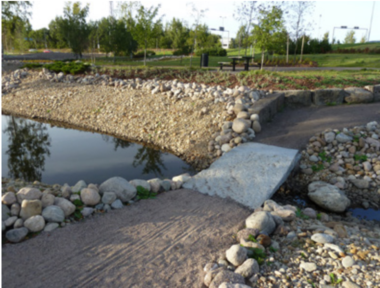
Figure 14. Cheek stones from a local stone processing factory are applied as bridges in the Saunarannanpuisto Park. Photo: Hannu Tolonen.
